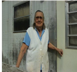
Patagonia resident, Lorena McKiddy, will have a dilapidated entryway replaced with a new platform and steps for safer access to her mobile home.
